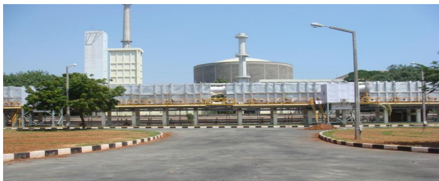
4.5 MLD MSF Plant at NDDP, Kalpakkam coupled to MAPS
